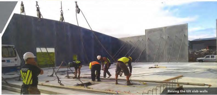
Raising the tilt slab walls
